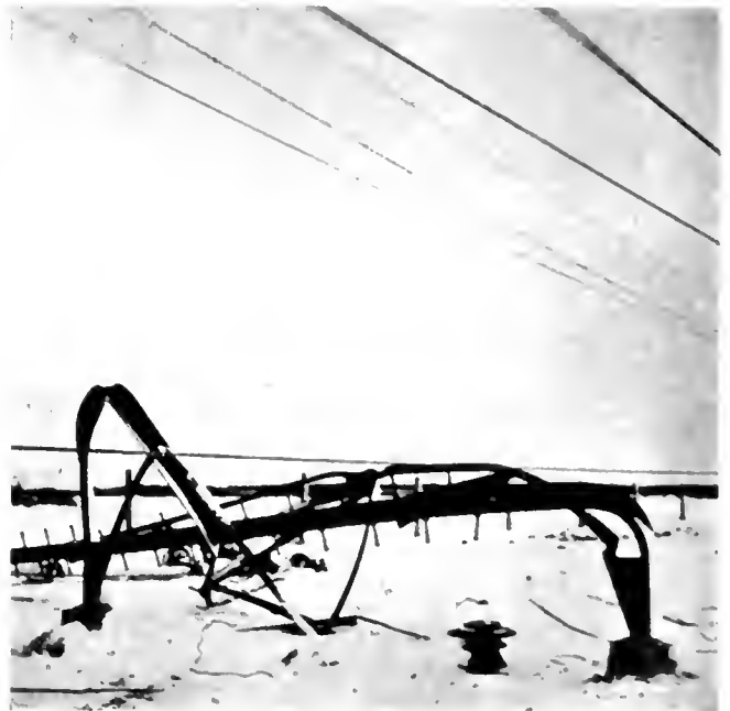
Sleet storm doubles up one of Winnipeg municipal towers.
